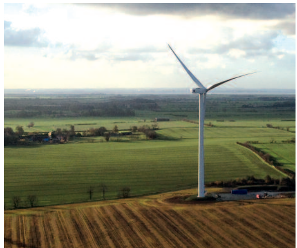
Windpark Burton Pidsea in England
